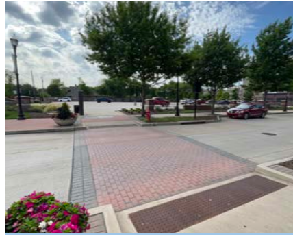
PEDESTRIAN SAFETY CROSSING
