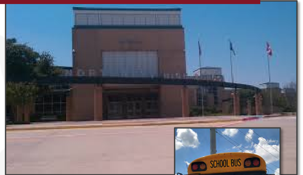
Northwest High School Addition and Renovation
