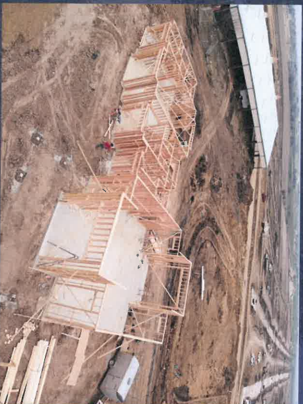
Building Framing Progress (February 2019)
